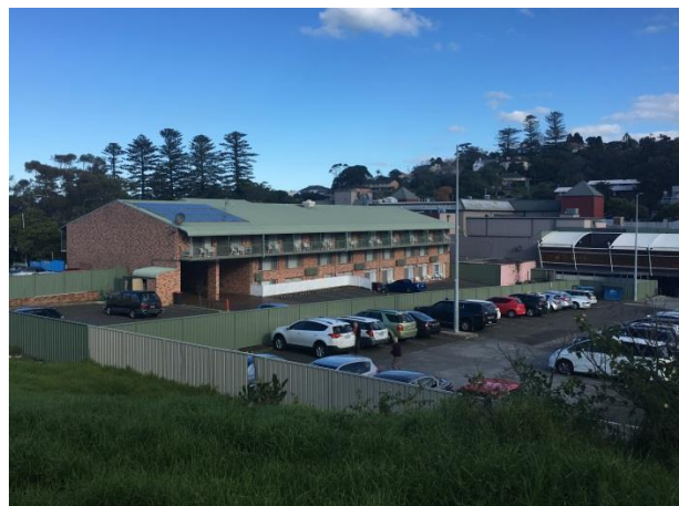
Picture 8 – Kiama Shores Motel and Leagues Club Carpark located to the south of the site
